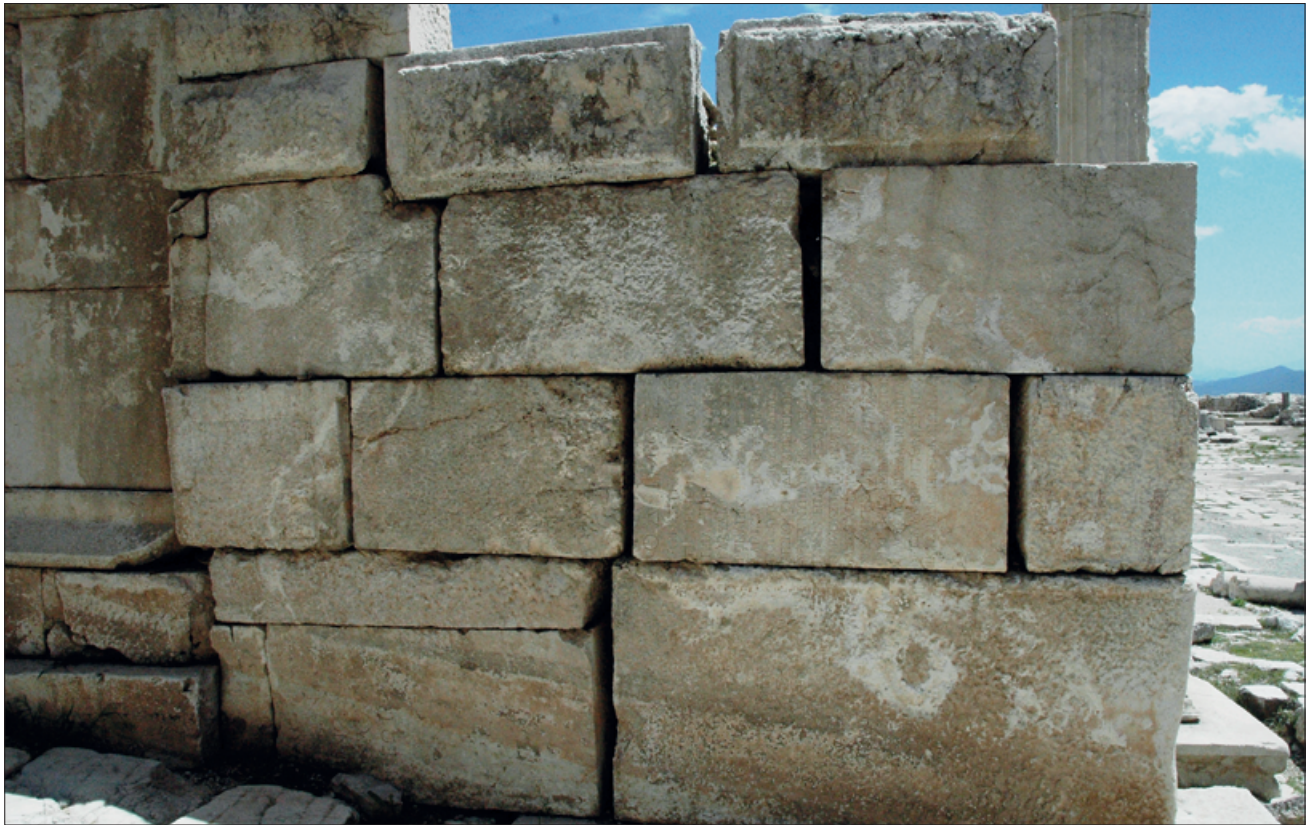
Fig. 14 North wall of North-East Building including reused elements of honorific monuments. – (Photo P. Talloen).
