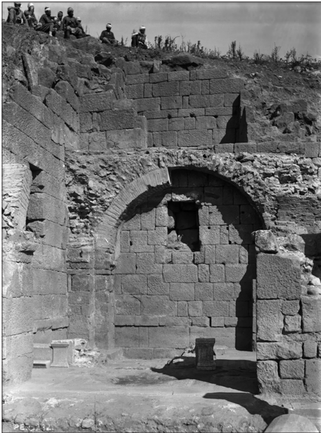
Fig. 5 Pergamon, Lower Agora. Northwestern corner with secondary piers, cross-vault and bema . – (Photo DAI, Neg.-Nr. D-DAI-ATH-Pergamon_0232).
