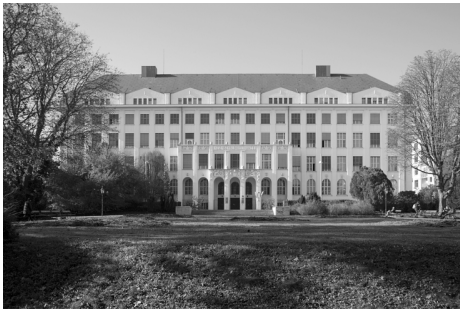
2. The building in Franz Klein-Gasse 1 in Vienna.
