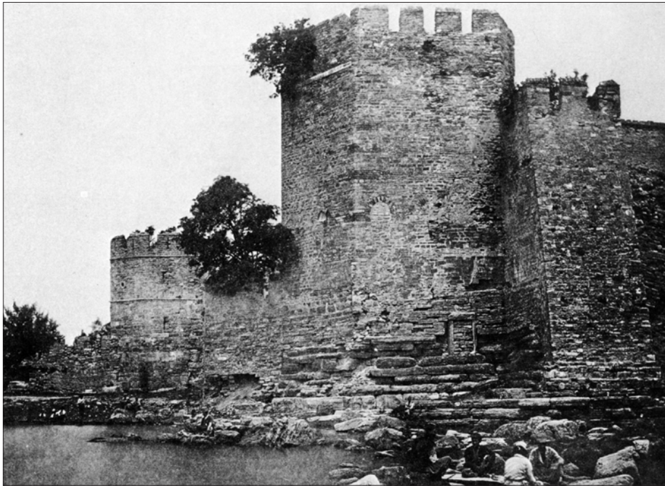
Fig. 9 The southern section of the Theodosian wall showing the external and internal walls, 1870s. – (From Meyer-Plath/Schneider, Landmauer pl. 25a).
