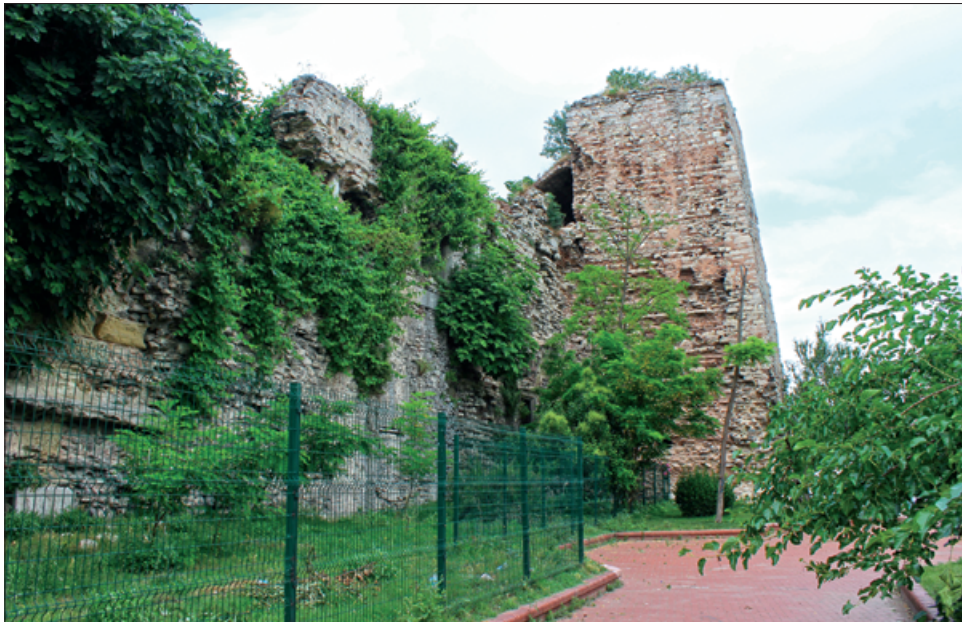
Fig. 26 The »lighthouse« on the sea wall today. – (Photograph G. Simonov 2016).
