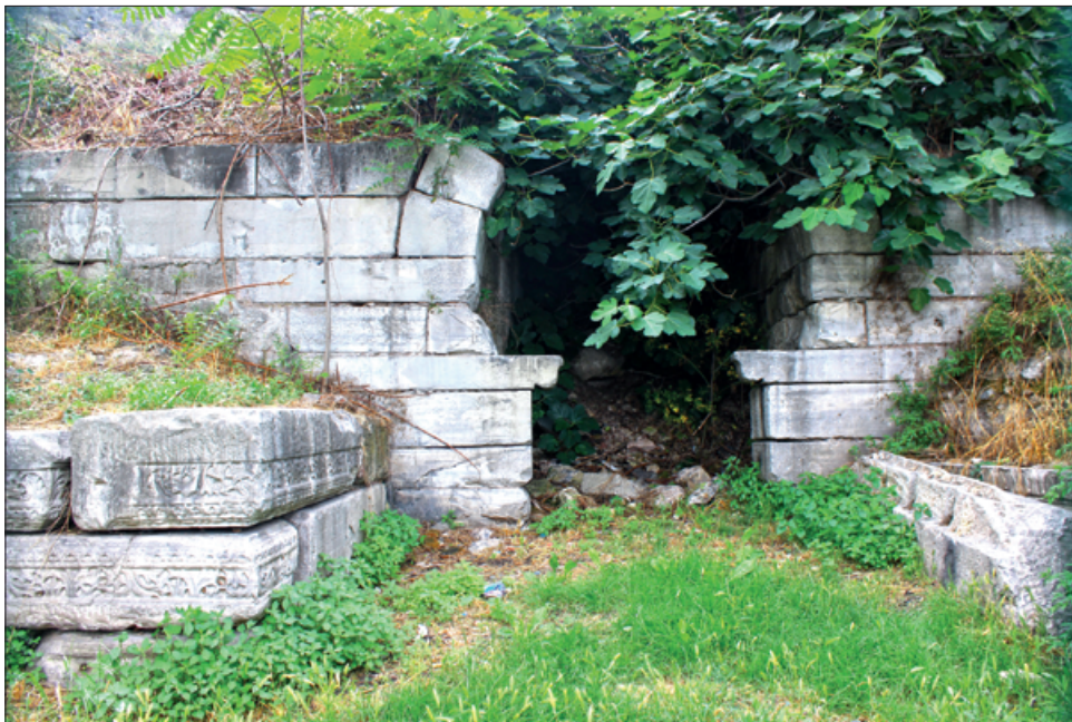
Fig. 19 The harbour portal Z2a/Z2b as it is today. – (Photograph G. Simonov 2016).
