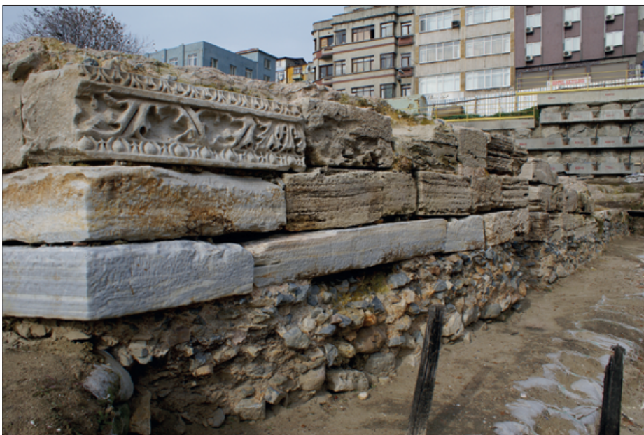
Fig. 5 Northern facade of the eastern jetty, Yenikapı. – (Photograph A. Ercan, from Ercan, Yenikapı 163).
