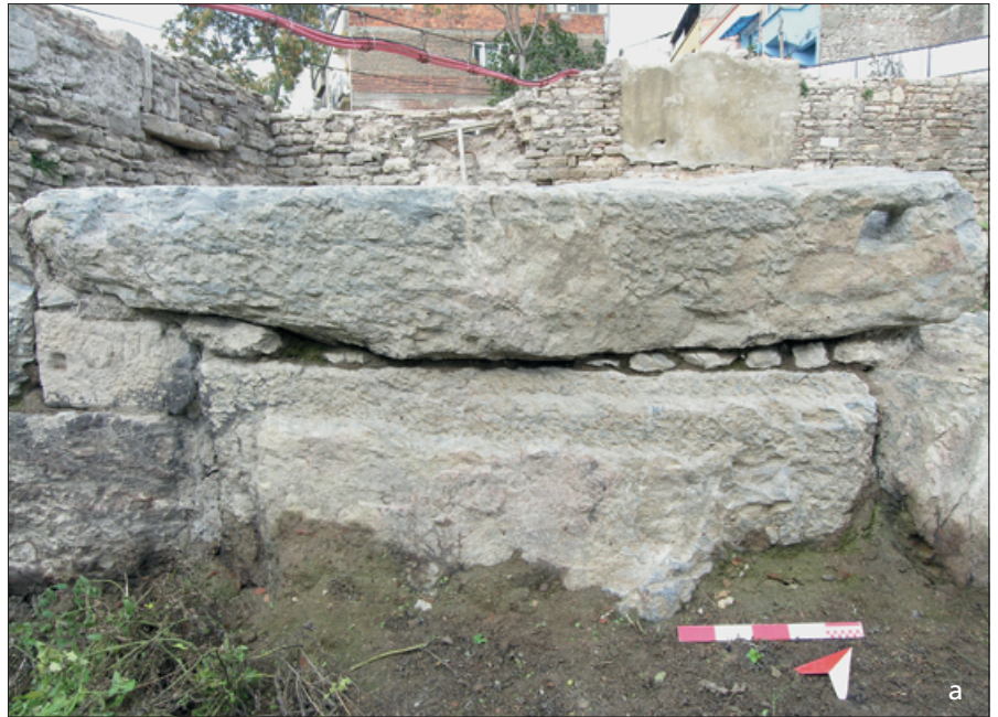
Fig. 29 a-b Yenikapı, spolia block and pierced stone block on the quayside. – c Jetty with pier extension in the Light Rail System Area north-west of Yenikapı excavation site. – (a-b photographs B. Köşker, IAM Archive; c from Kızıltan, İstanbul Kazıları 360).
