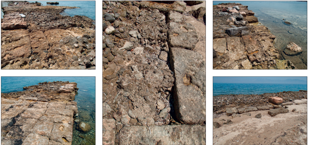
Fig. 14 Chamber system of the northern mole construction of the harbour of Anthedon. – (Photo A. Ginalis, 2018).
