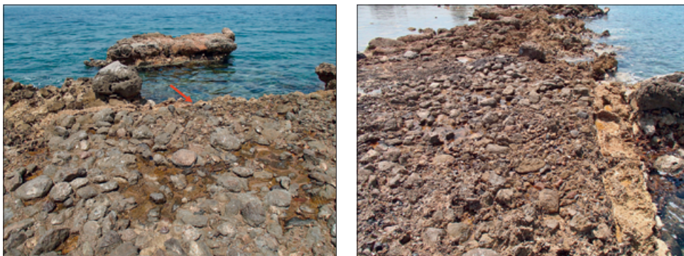
Fig. 16 Detail views of the northern mole construction of the harbour of Anthedon. – (Photo A. Ginalis, 2018).
