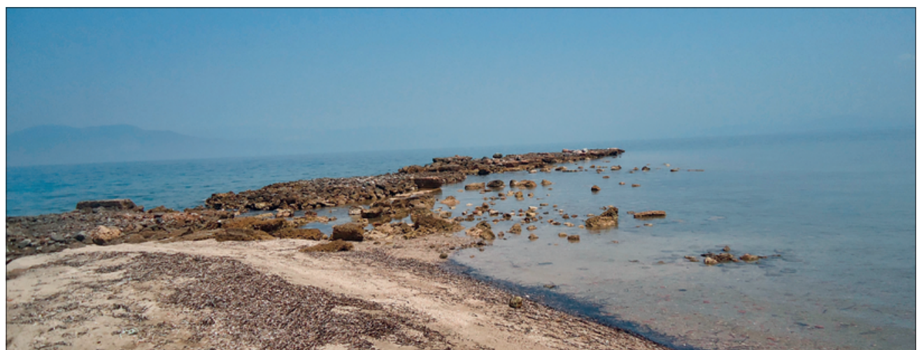
Fig. 13 Northern mole construction of the harbour of Anthedon. – (Photo A. Ginalis, 2018).
