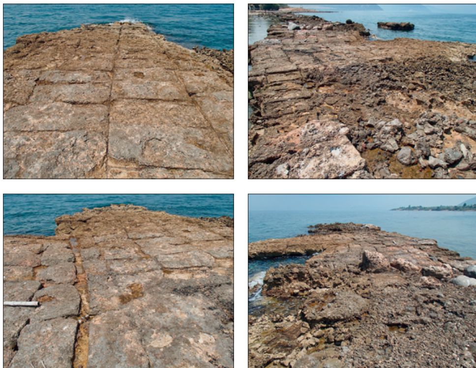
Fig. 17 Superstructures on the northern mole construction of the harbour of Anthedon. – (Photo A. Ginalis, 2018).
