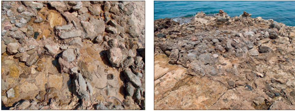
Fig. 15 Detail views of the northern mole construction of the harbour of Anthedon. – (Photo A. Ginalis, 2018).
