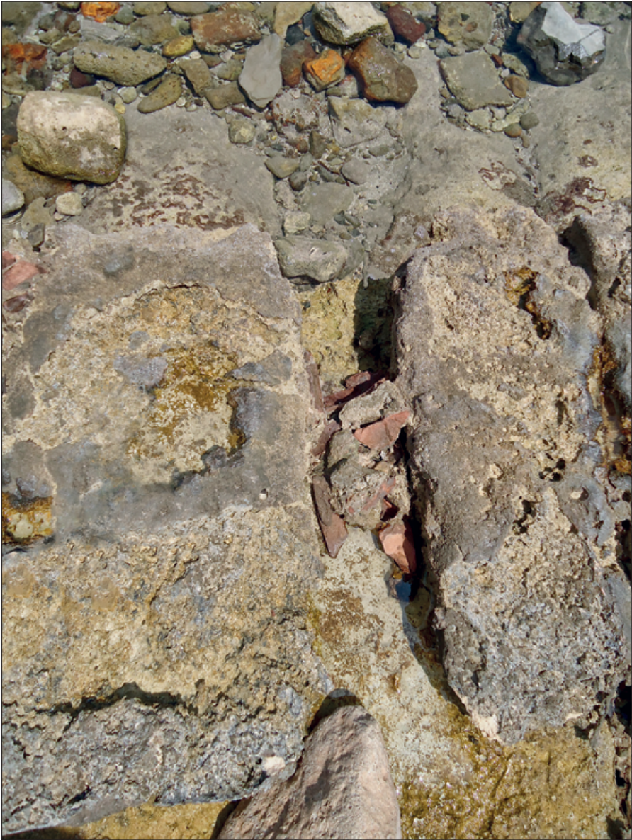
Fig. 35 Detail views of the southern quay of the harbour of Anthedon. – (Photo A. Ginalis, 2018).
