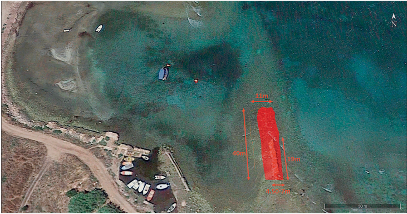
Fig. 22 Measures of the eastern mole construction of the harbour of Anthedon. – (Photo A. Ginalis, 2018).
