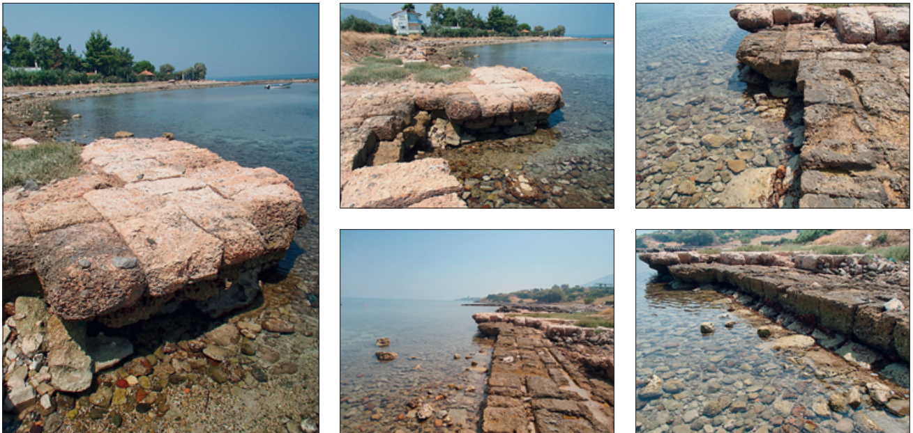
Fig. 32 Jetty-like platform in the southern quay of the harbour of Anthedon. – (Photo A. Ginalis, 2018).
