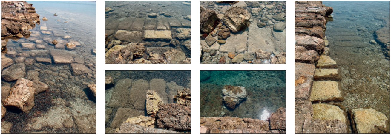
Fig. 12 Stone layer at the inner side of the breakwaters of the harbour of Anthedon. – (Photo A. Ginalis, 2018).
