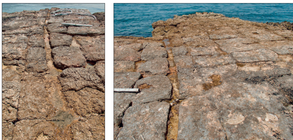
Fig. 18 Superstructures on the northern mole construction of the harbour of Anthedon. – (Photo A. Ginalis, 2018).
