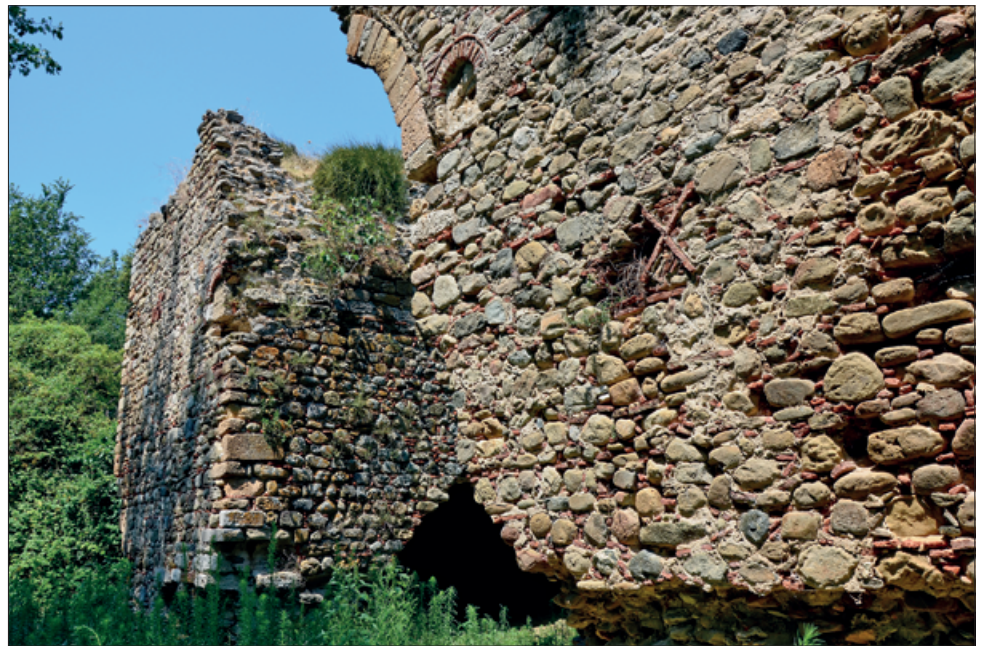
Fig. 11 Anastasioupolis. Harbour gate from north-east. – (Photo Th. Schmidts).
