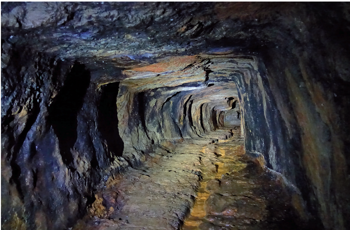
Fig. 7: Territorium metallorum Tresminas/Jales: The Galeria dos Morcegos with pilot drift and partial excavation.
