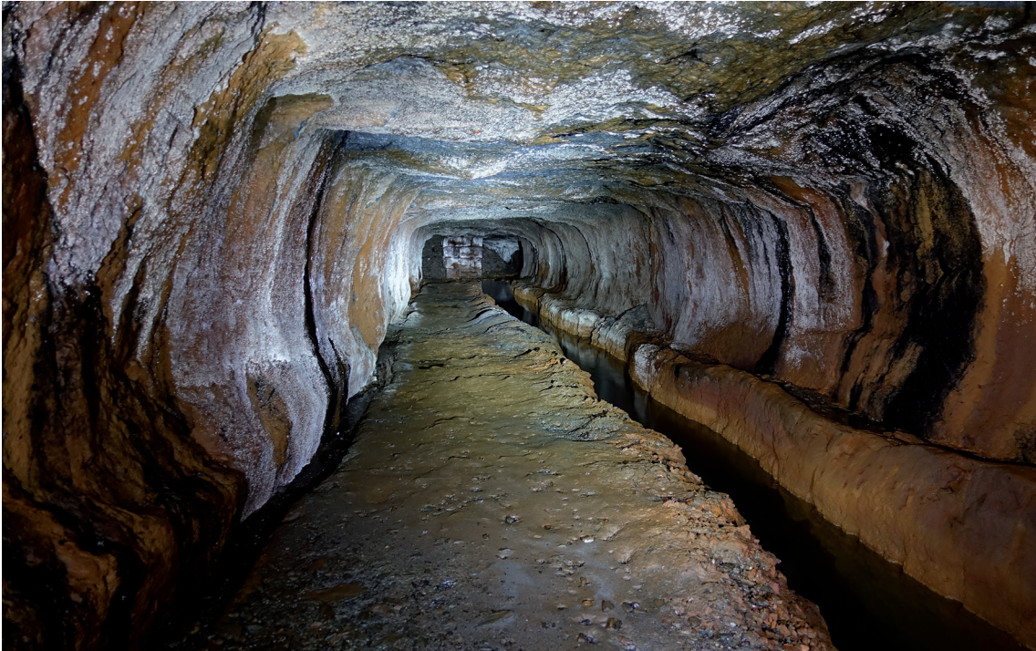
Fig. 3: Territorium metallorum Tresminas/Jales: Galeria do Pilar with the channel (0.8–1 m wide and 23 m deep) and the pillar that gave it its name in the background.
