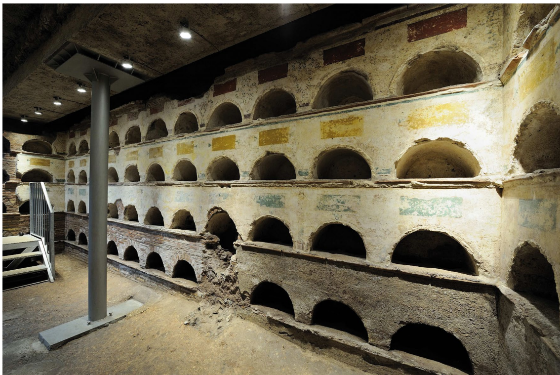
Fig. 3: General view of the South wall of the columbarium A. AF-MonAS – MSCD 145-434.
