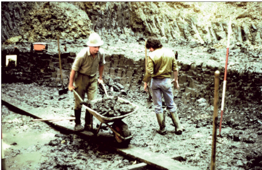
Fig. 7 Excavators clear the soil and rocky material above the site in 1985. The dark grey clay of the bone bearing layer is cut at a depth of approximately 2 m below the person standing in the centre of the picture. – (Photo: Natural History and Mammoth Museum Siegsdorf).
