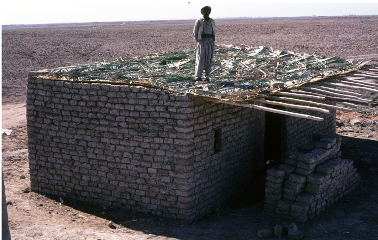
Fig. 4. Making a roof – Abu Salabikh 1976. Photo by the author.
