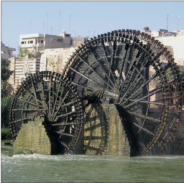
Fig. 1 Noria water-lifting wheels, originally constructed in early Islamic times. Hama on-the-Orontes River. – (Photo K. D. Politis).
