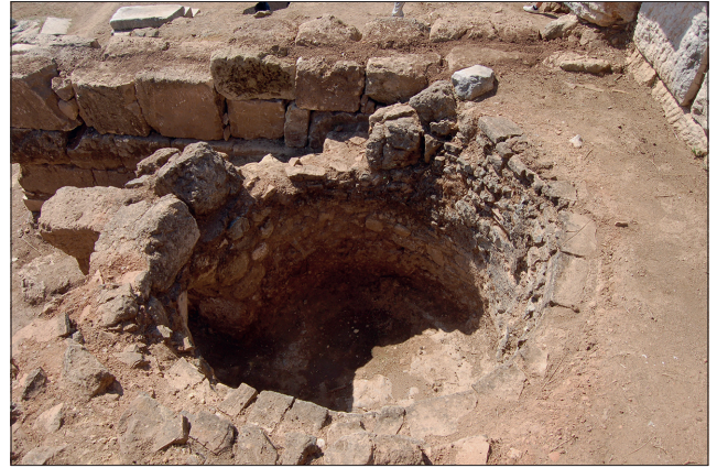
Fig. 7 Messene, Early Byzantine lime-kiln in the theater's outer wall, view from North – (Photo Society of Messenian Archaeological Studies).
