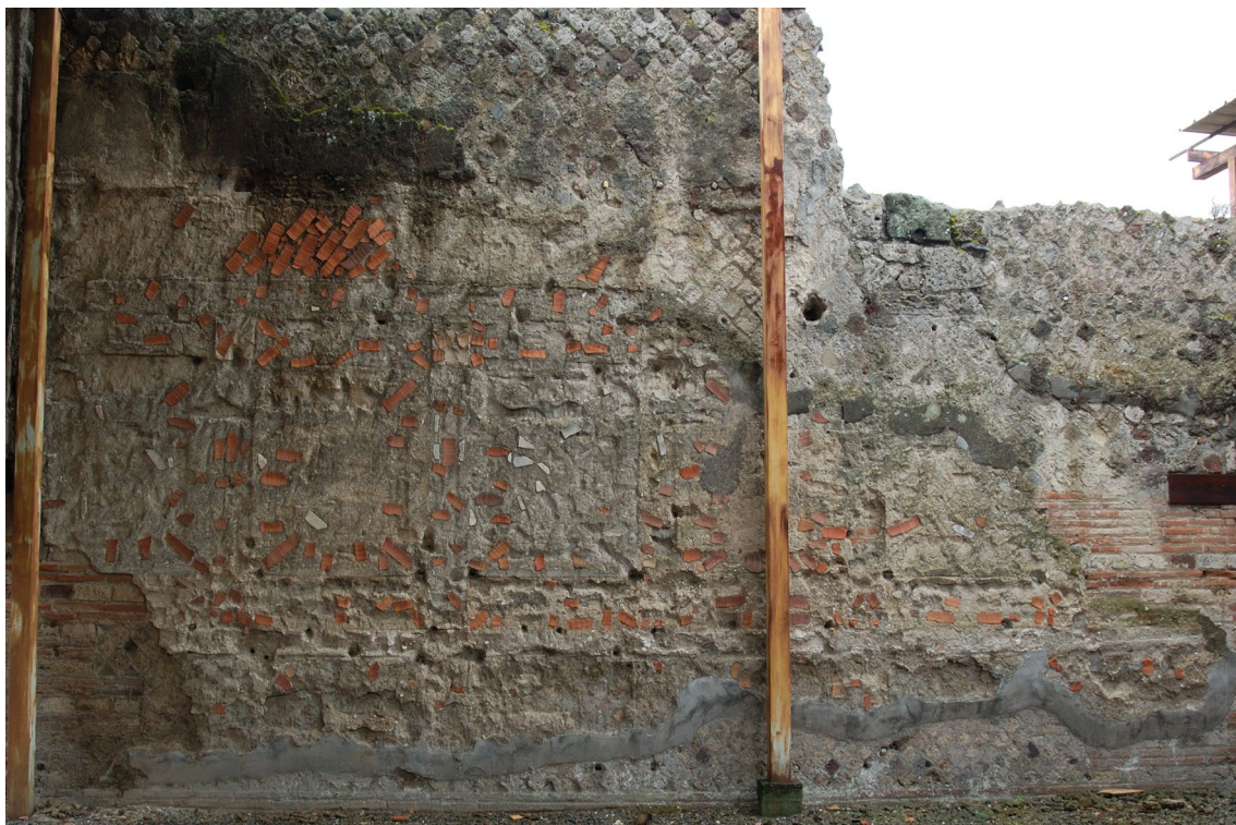
Fig. 6: Pompeii, House of Dioscuri, room 46, example of a preparatory layer for a (stripped) marble veneer.
