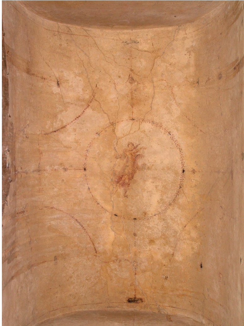
Fig. 2: Rome, Domus Flavia, room 334, vault.
