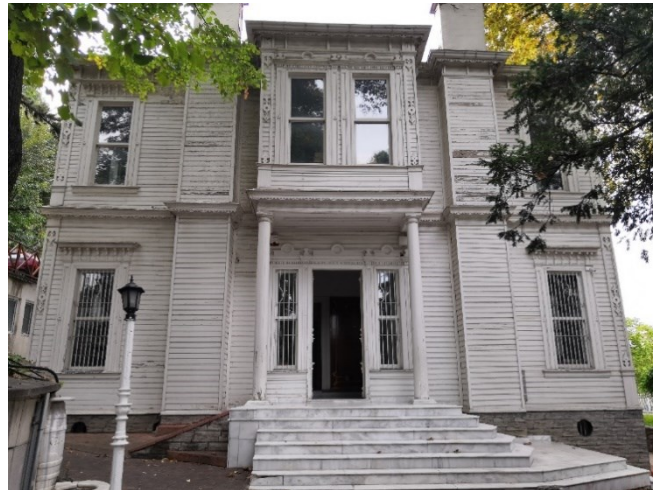
Fig. 2. Southeastern Façade of the Building and the Main Entrance, Bursa, Turkey (© Oğuz Yeke).
