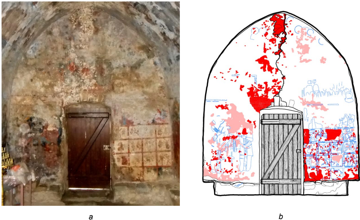
Fig. 6. West internal façade a) Orthophoto b) AutoCAD drawing with pathology mapping.
