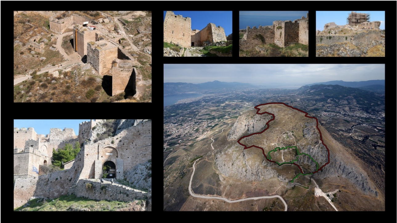
Fig. 5. Aerial Photos & signalization of the main Walls of Acrocorinthos Castle (© IMANTOSIS [2014]).
