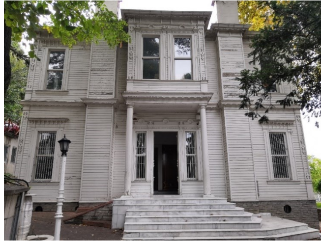
Fig. 2. Southeastern Façade of the Building and the Main Entrance, Bursa, Turkey (© Oğuz Yeke).
