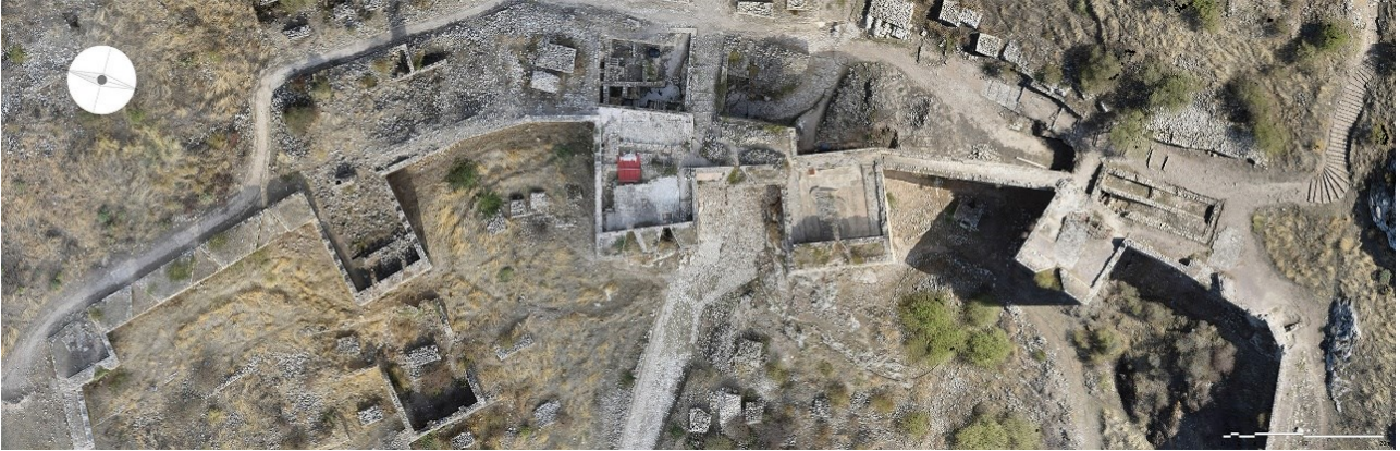
Fig. 9. Orthophotomosaic / Part of West Fortification of Acrocorinthos Castle (© IMANTOSIS [2014]). Details of original Orthophotomosaic: accuracy 1cm / pixel size 3 mm / 50 artificial ground targets (GCPs) & more than 400 physical targets all measured by total station. Processed & Produced in Agisoft Photoscan Software.
