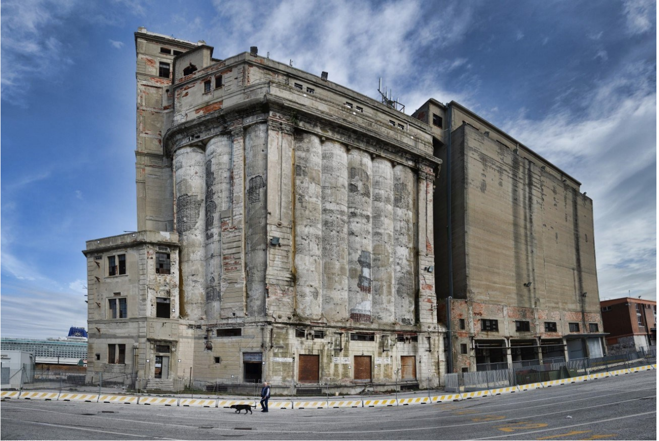
Fig. 2. The Silos in 2019 (© Authors).
