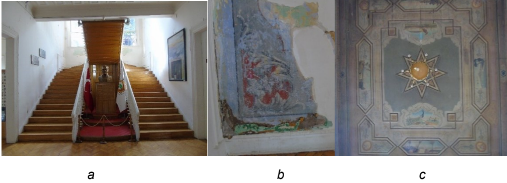
Fig. 3. Forestry Museum inner walls and ceiling ornaments. a) Stair Hall; b) Ornament in Stair Hall Wall; c) Room Ceiling Detail (© Oğuz Yeke).
