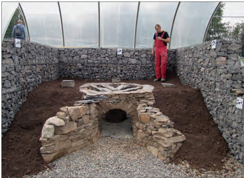
Fig. 3 Unlike the original discovery, the test kiln was not embedded in an existing hillside. It was set up in a gabion in the open and then backfilled with sediment. In this way, the sample chambers for the thermocouples could also be erected next to the furnace wall. – (Photo RGZM).
