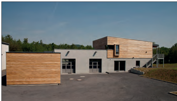
Fig. 6 The Labor für Experimentelle Archäologie of the RGZM in the Mayen mining area. – (Photo B. Streubel, RGZM).
