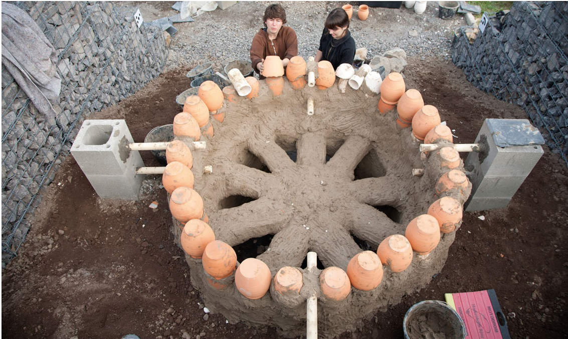
Fig. 2: Construction of the firing chamber using upside down pots.
