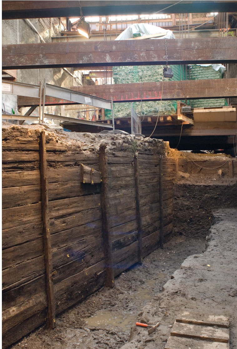
Fig. 9: Cologne, Kurt-Hackenberg-Platz. Wooden shuttering from the foundation of the Roman town wall.
