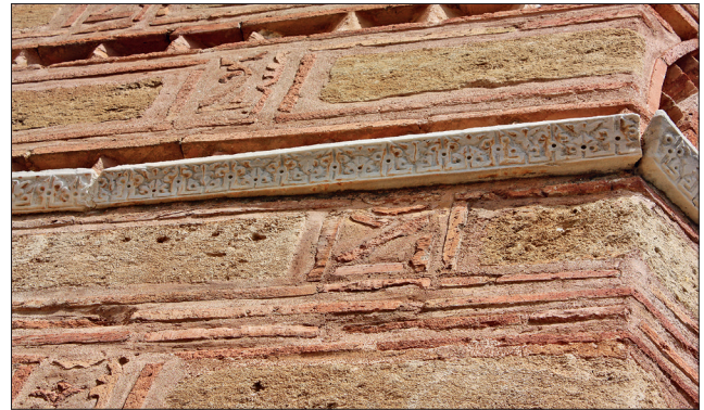
Fig. 6 Pseudo-Arabic carved marble string course, east façade, Hosios Loukas, ca. 961. – (Photo A. Walker).
