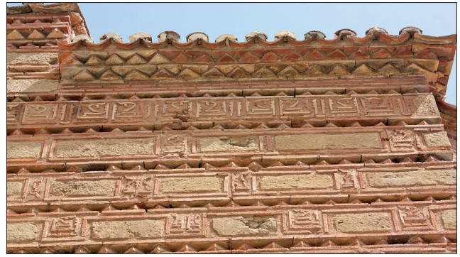
Fig. 5 Pseudo-Arabic cloisonné bricks, east end of south wall, Hosios Loukas, ca. 961. – (Photo A. Walker).
