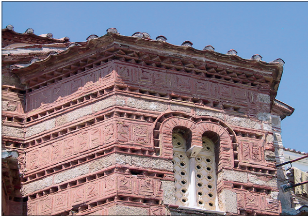
Fig. 3 Pseudo-Arabic cloisonné bricks, central apse, east façade, Hosios Loukas, ca. 961. – (Photo A. Walker).
