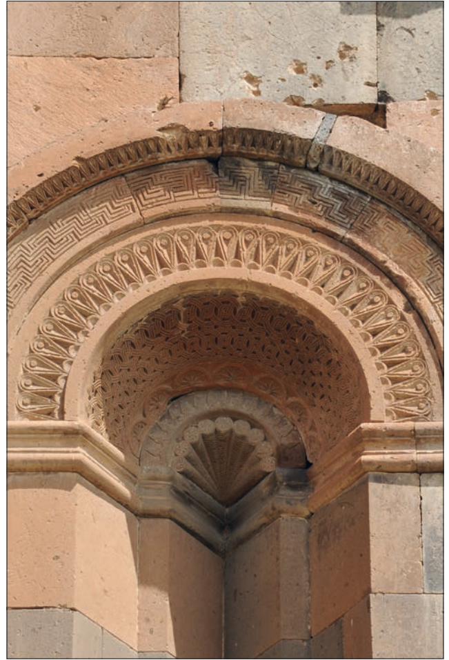
Fig. 12 Ani, Cathedral, southern facade: squinch of the niche. – (Photo A. Kazaryan / L. Mikayelyan).
