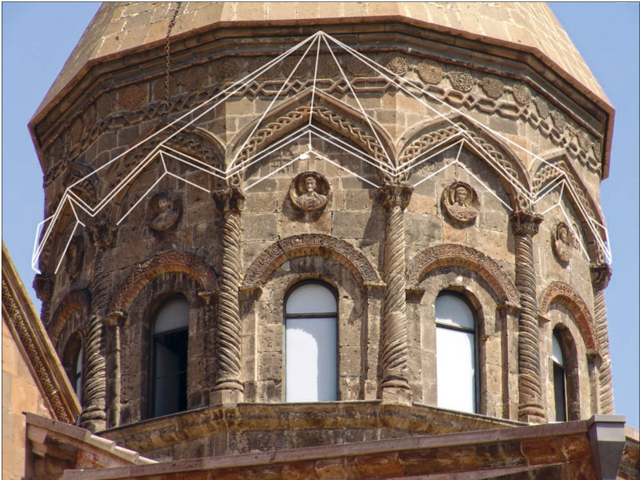
Fig. 5 Vaghharshapat, Etchmiadzin Cathedral, drum (ca. 620): reconstruction by A. Kazaryan 2007. – (Photo A. Kazaryan / L. Mikayelyan).
