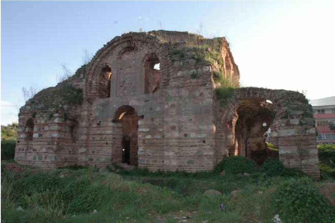
Church of Saint Averkios Gemlik county, Kurşunlu neighborhood, Çatal locale
