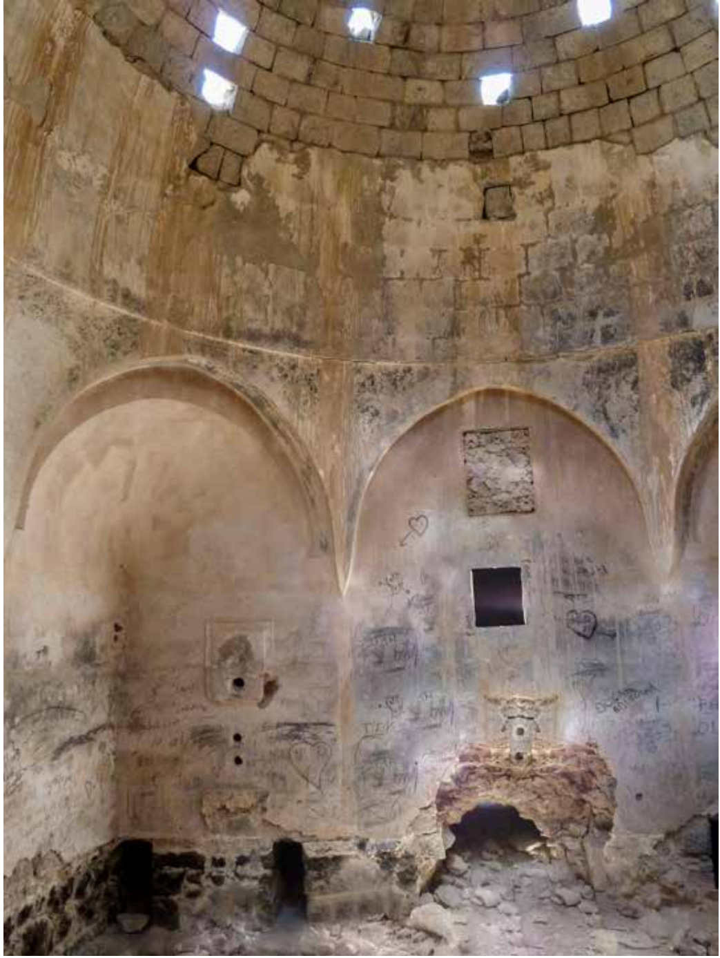
The Public Bath Niğde Central county, Yeşilburç village
