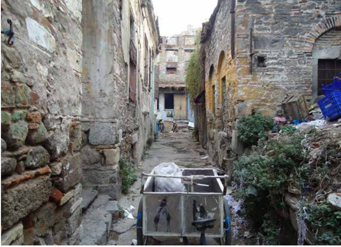
Cortijo structure no.5 (Taş Cortijo) Residential units surrounding the street
