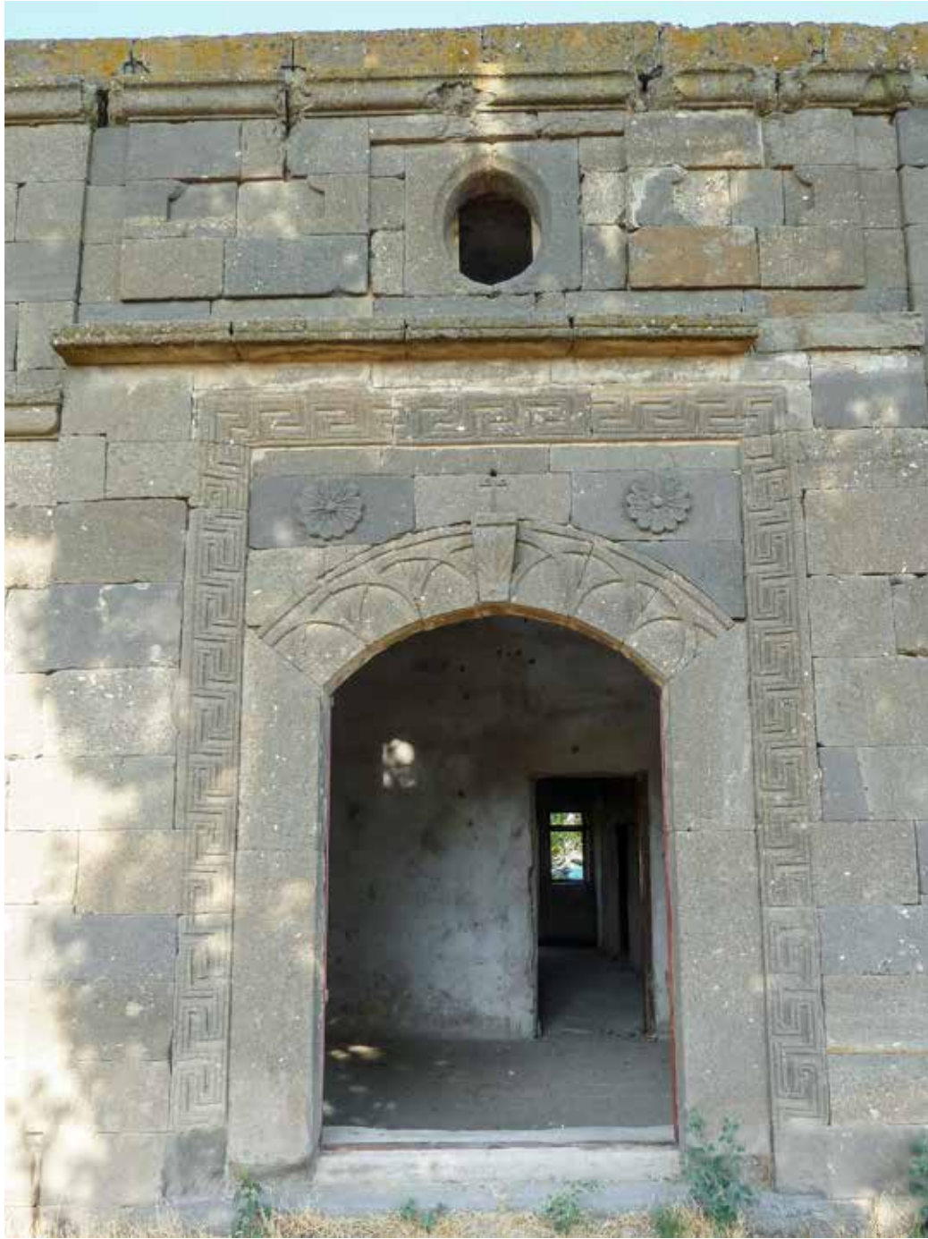
The Greek School Niğde Central county, Hasaköy neighborhood, Köyiçi locale
