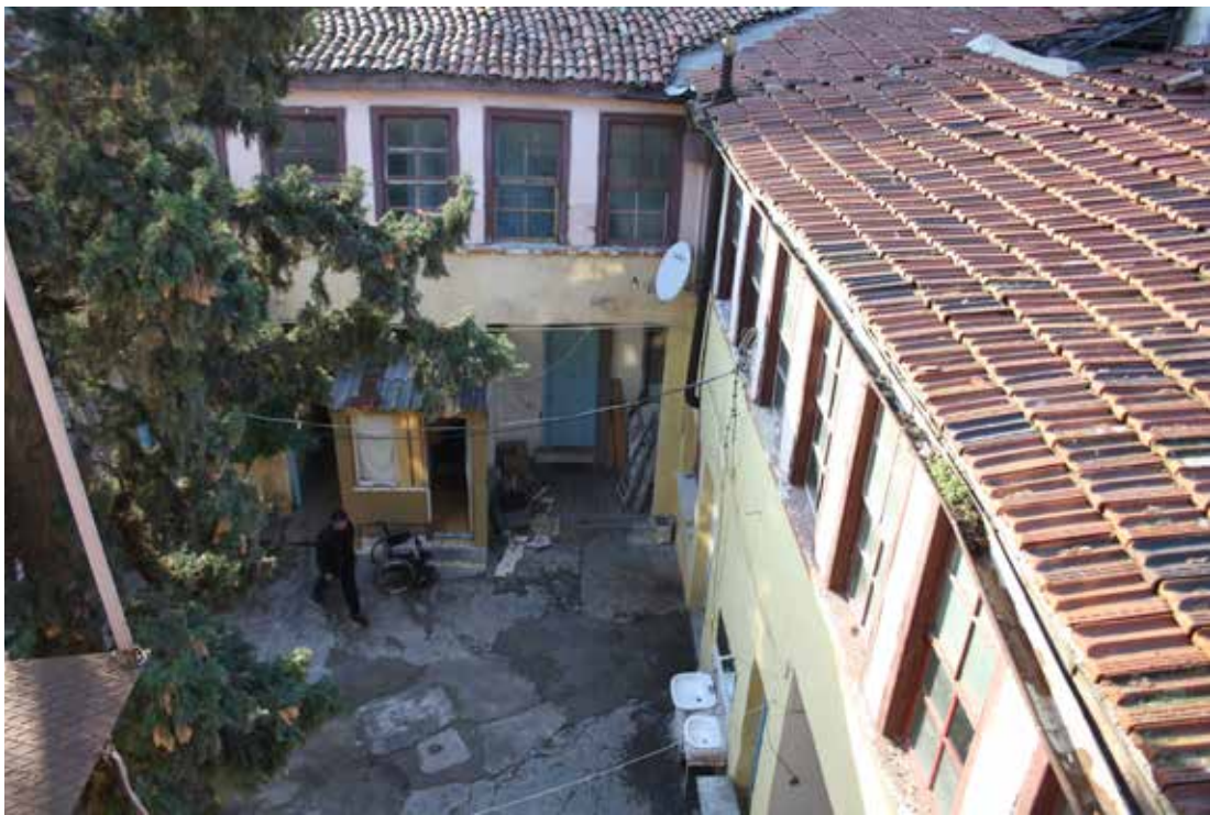
Cortijo structure no.1 Courtyard and blocks opening to the courtyard
