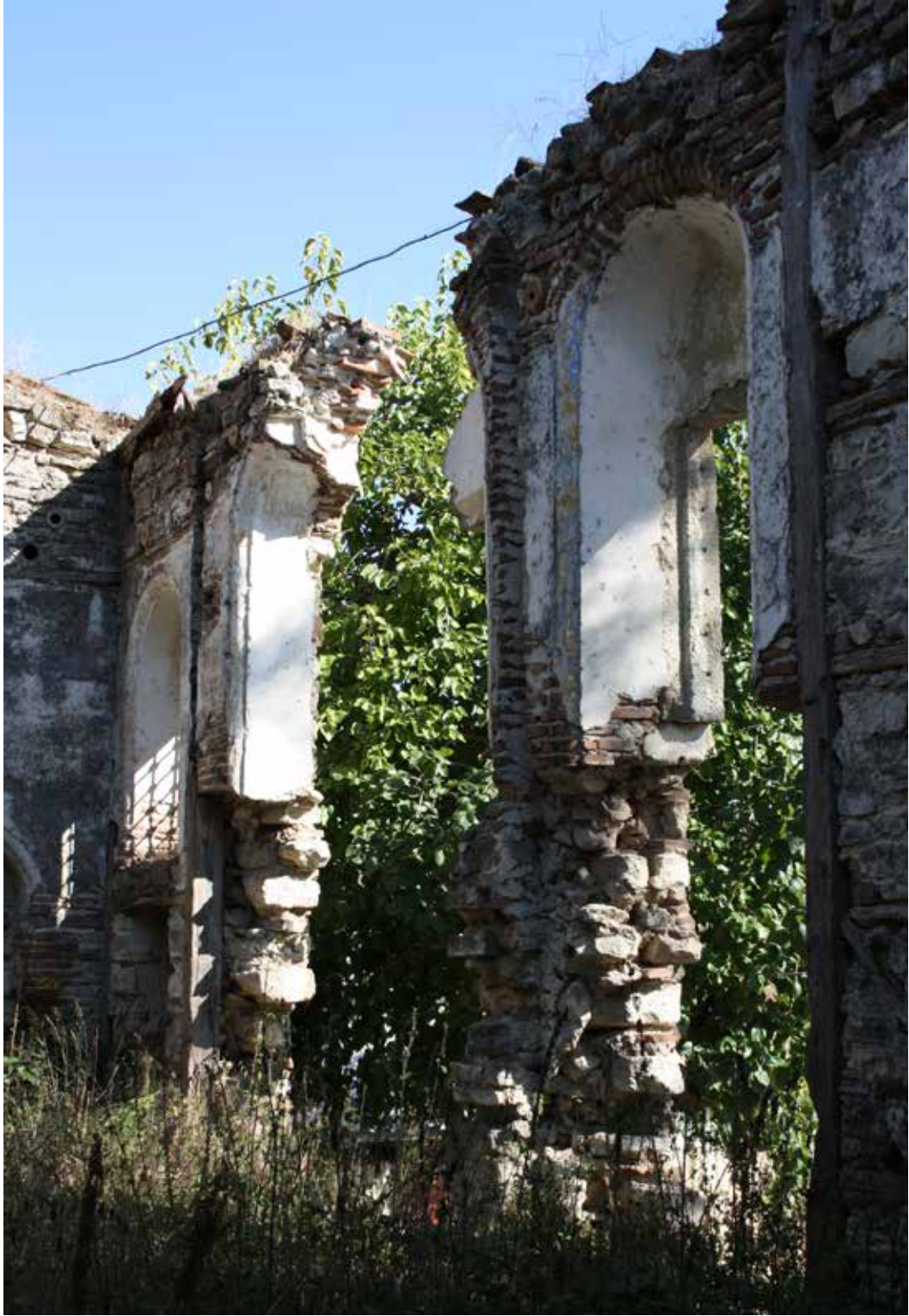
Church of Saint George Karacabey county, Çamlıca neighborhood
