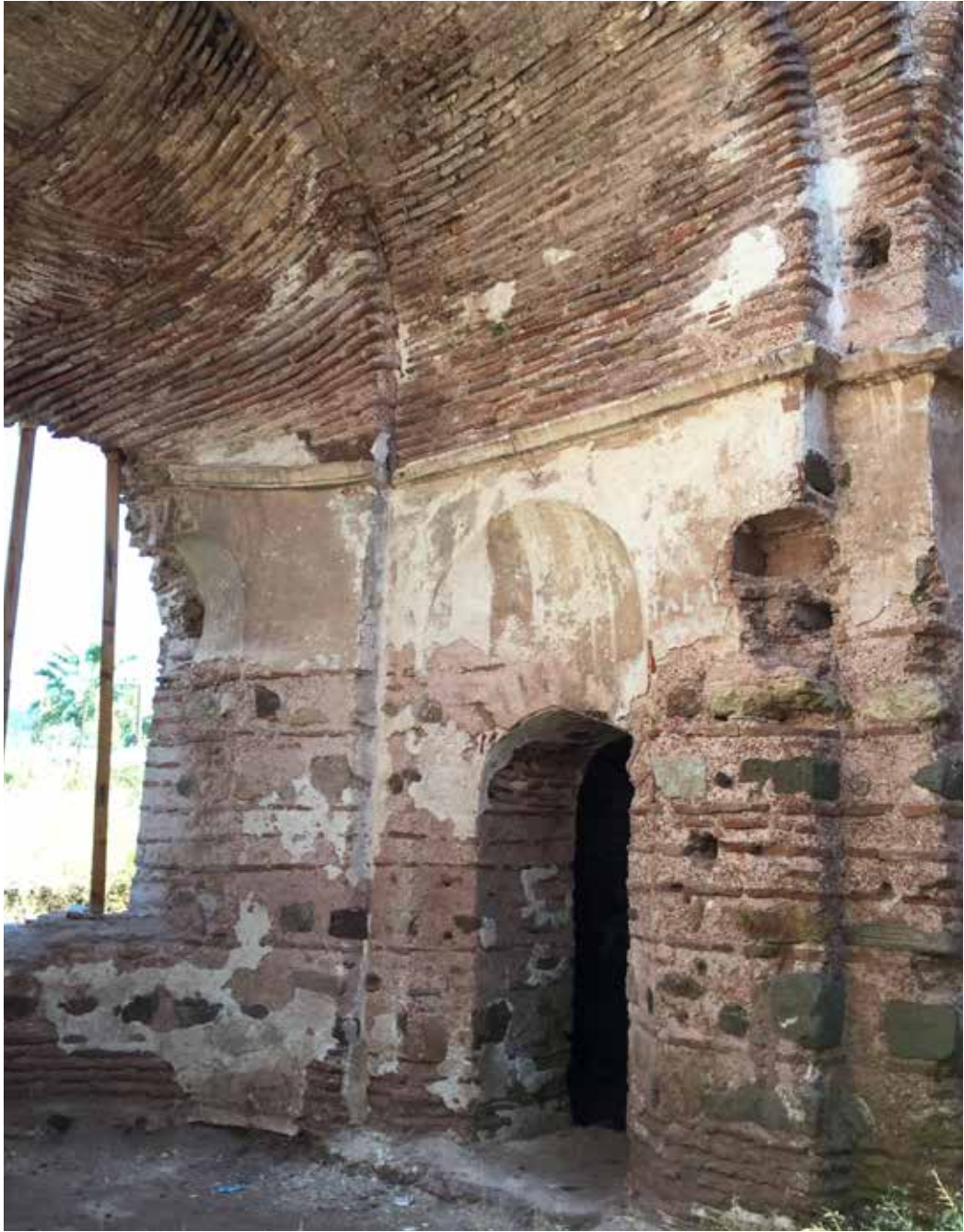
Church of Saint Averkios Gemlik county, Kurşunlu neighborhood, Çatal locale
