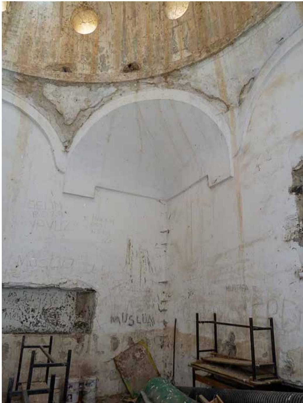
dome. There is no longer any glass in the skylights. The passage from the structure into the barrel-vaulted water tank is through a window in the western wall of the hot section. The existence of a buried hearth in the furnace section is hinted at by an arch southwest of the structure. The hamam is very sparse in terms of decoration due to being both very functional and located in a
