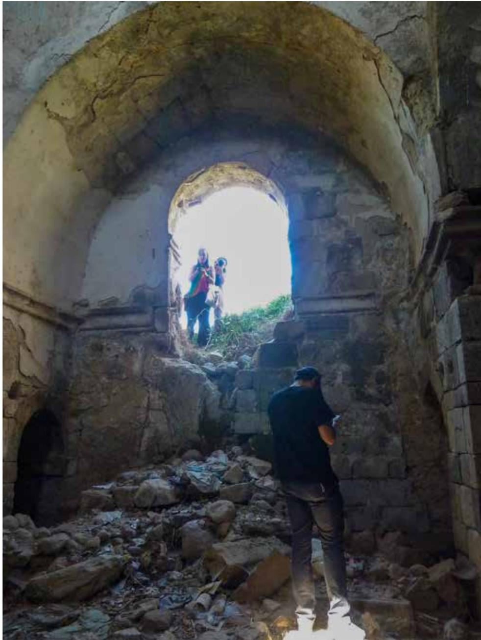
The eastern bay, which served as the bema, ends in a horseshoe shaped apse (4.3 m in width and 3.29 m in length) crowned by a half-dome, 2.85 m in height; it is flanked by two small niches. The apse is roofed in its lower part by large blocks in a horizontal direction; its inner surface is circular, and the outer one is pentagonal, with three axially placed openings at the lower part.
