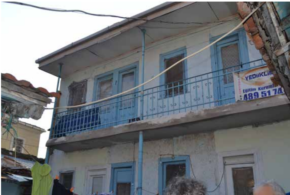
Cortijo structure no.4 Two floor block
