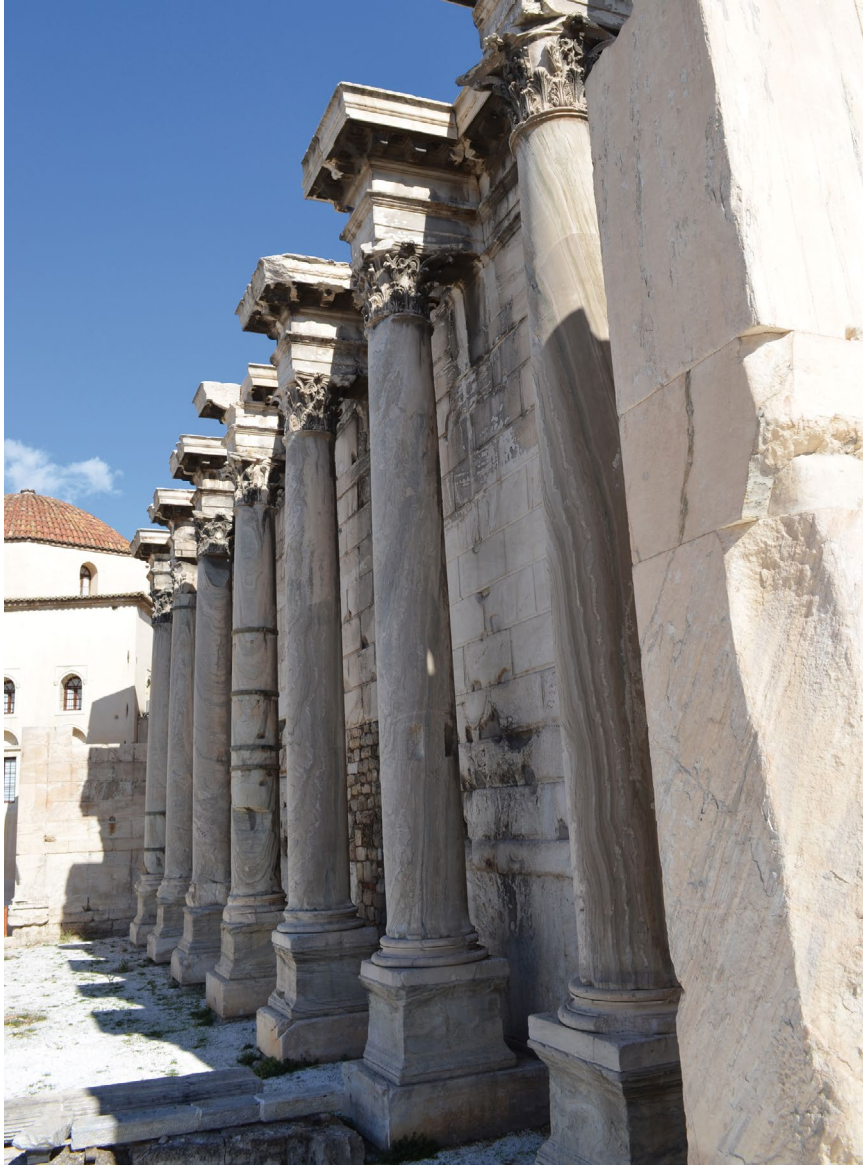
Fig. 7: Athens, Hadrian's Library, western colonnade outside the enclosure with Cipollino marble pedestals.
