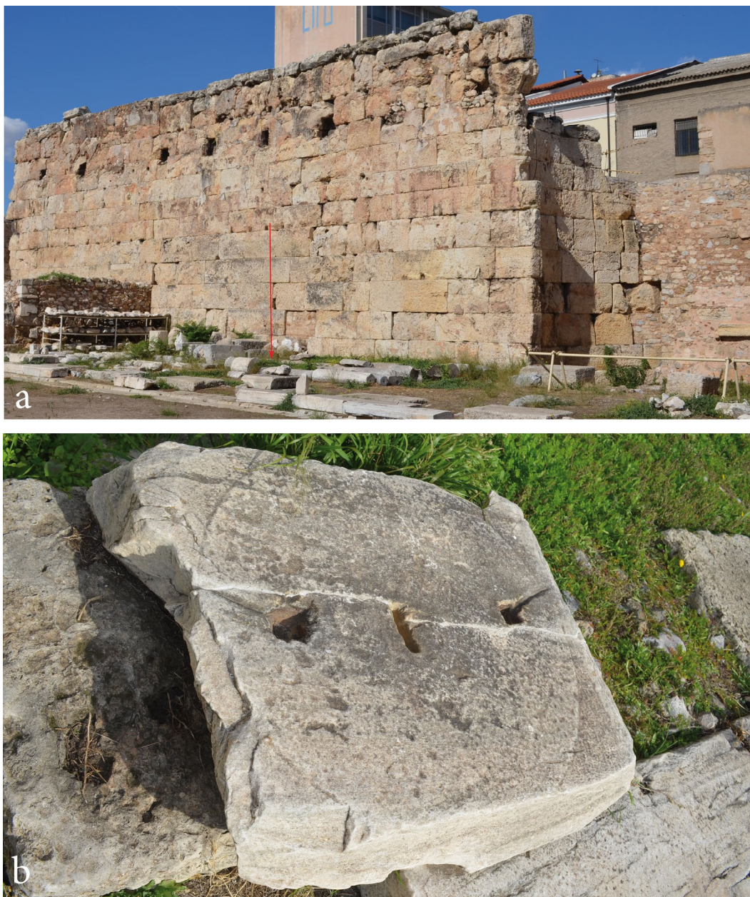
Fig. 5: Athens, Hadrian's Library, northern portico; a: position of one of the surviving stylobate slabs; b: slab of the stylobate with a circular carving.
