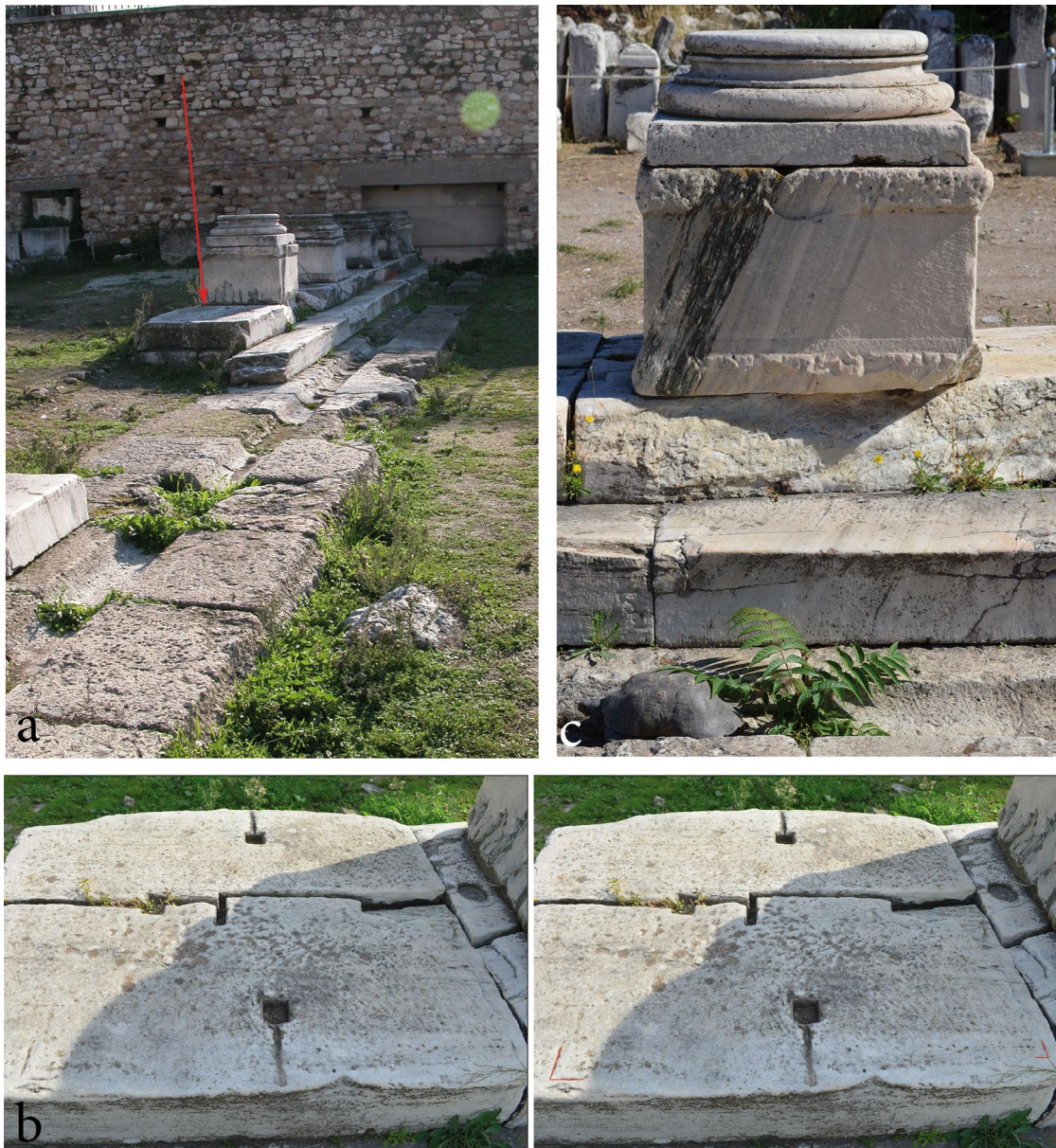
Fig. 6: Athens, Hadrian's Library, western portico; a: position of one of the stylobate slabs with angular carving lines; b: the stylobate slab with engraved the angles for the placement of square-based object; c: a plinth preserved in situ .
