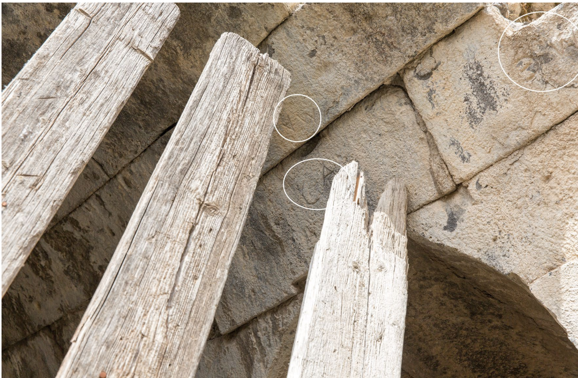
Fig. 4: Masons' mark documented on the vault of one of the passages of the Western Theatre of Gadara.
