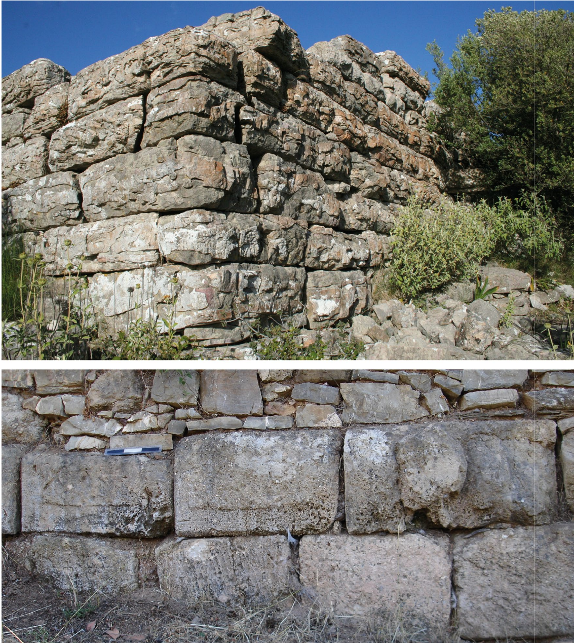
Figs. 4: a. Messene. West corner of T 24 built of hard limestone of mediocre quality with inclusions. b. Remains of the outer face of the psammite curtain south of the West Gate.
