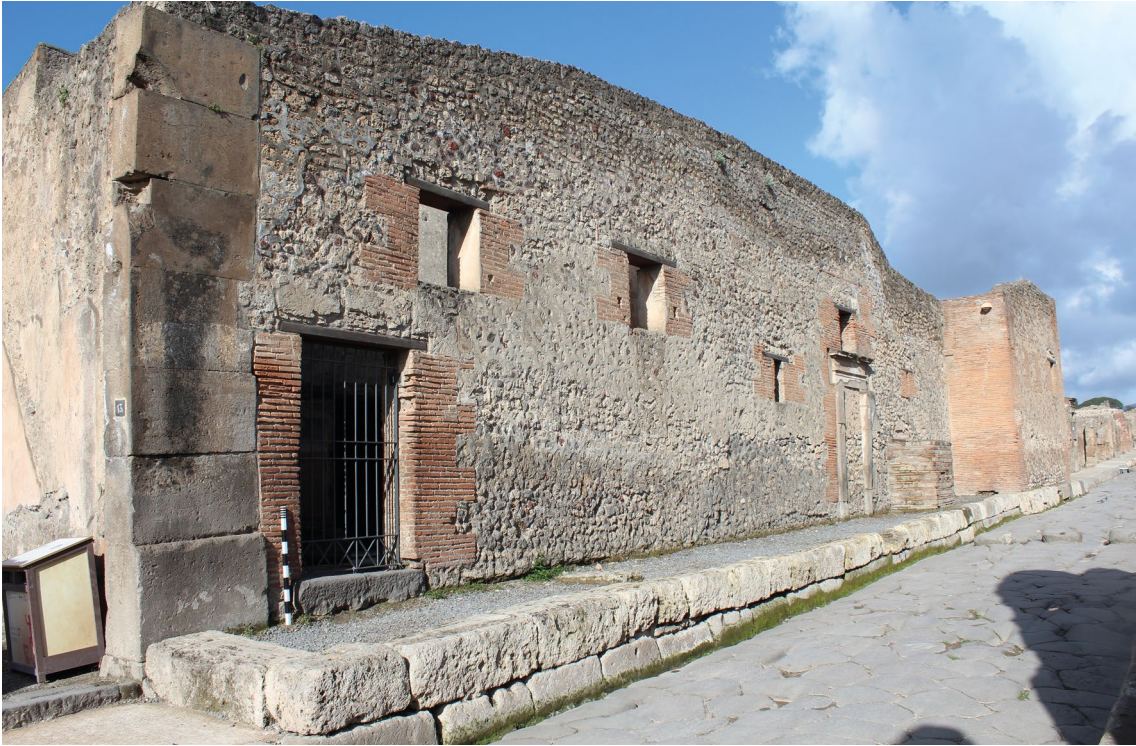
Fig. 6: Stabian Baths, E façade rebuilt after AD 62 with frames of fired bricks, from SE.
