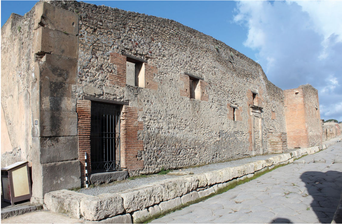
Fig. 6: Stabian Baths, E façade rebuilt after AD 62 with frames of fired bricks, from SE.
