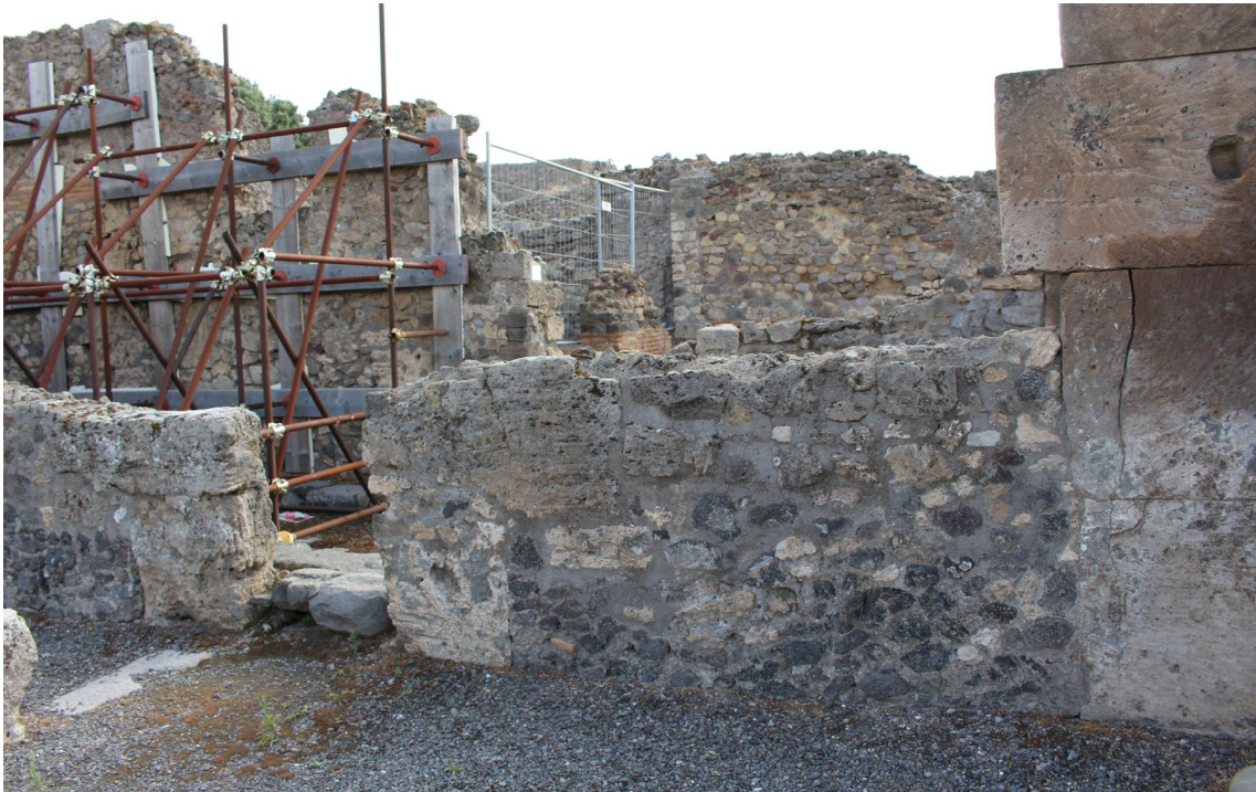
Fig. 2: Typical wall of opus incertum with lava and limestone ( taberna VIII 5, 20).
