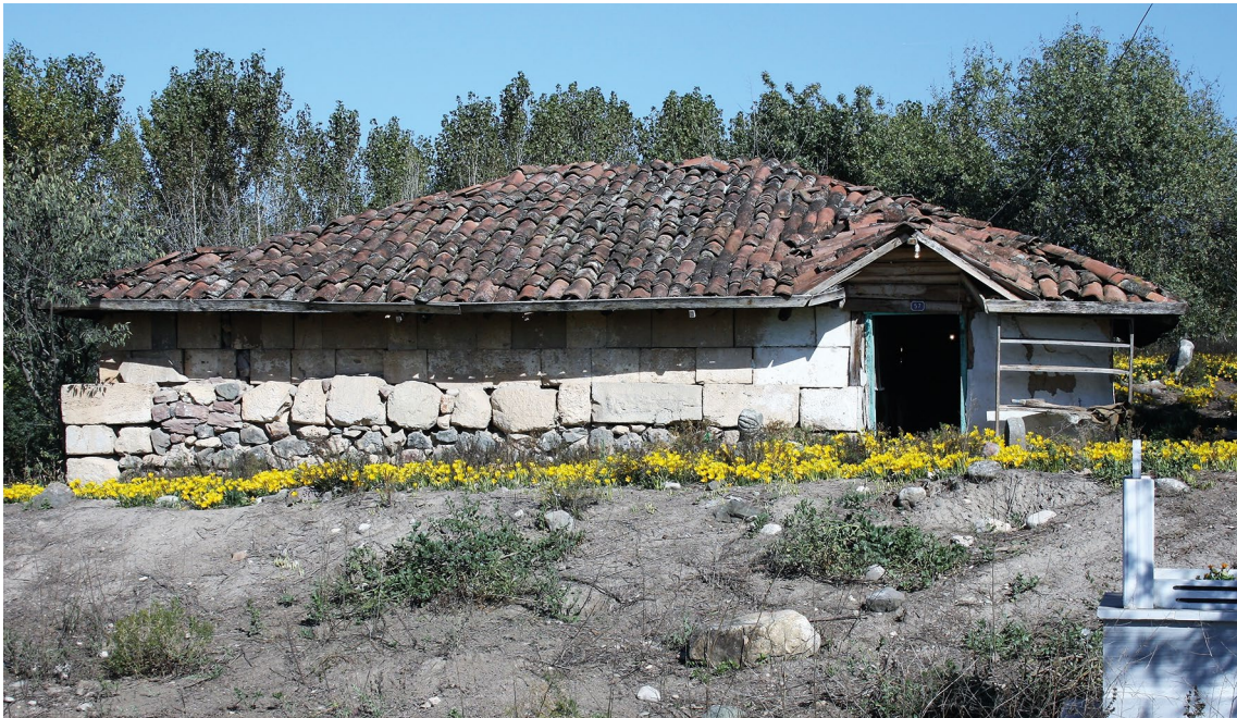
Fig. 4: This türbe in the cemetery of Çevresu rests on a foundation of large, regular stone blocks, possibly the remnants of a Roman structure.
