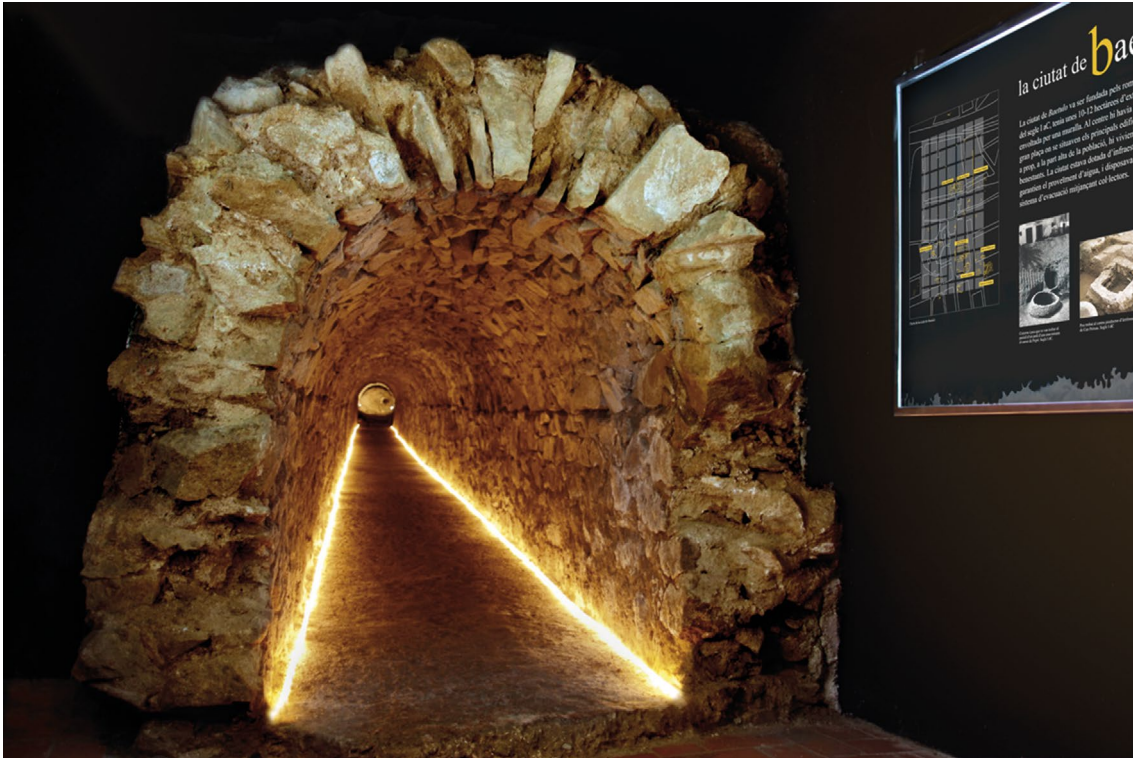
Fig. 2: Water conduct. Pujol Street.
