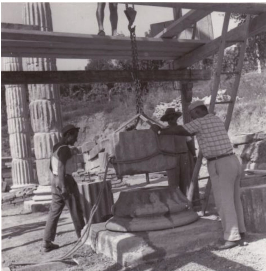
Fig. 3: The reconstruction of the columns of the main porticus.
