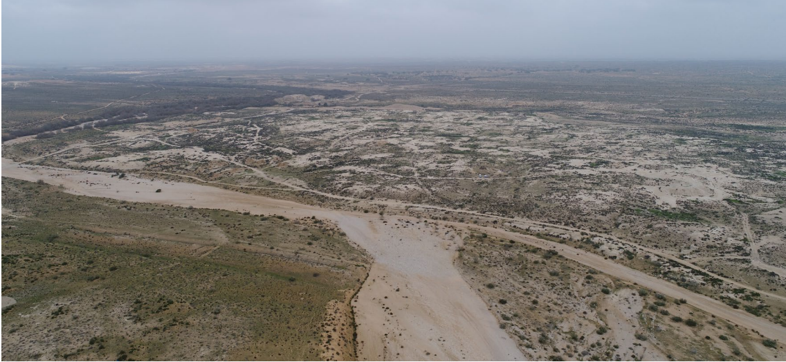
Fig. 2: Elusa. Aerial overview from South.
