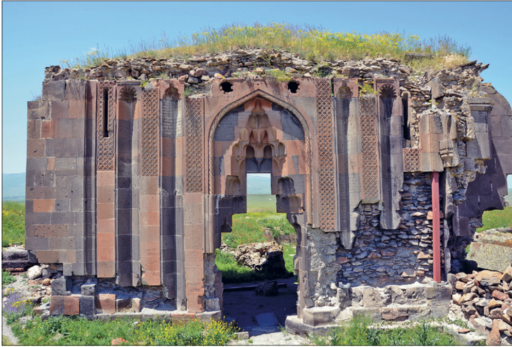
Fig. 10 Ani, church of the Holy Apostles. East façade of the gavit; ca. 1217. – (Photo A. Eastmond).
