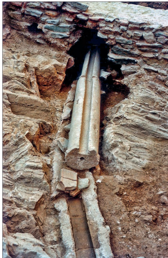
Fig. 355 7 Glaukou Street, water pipe.
