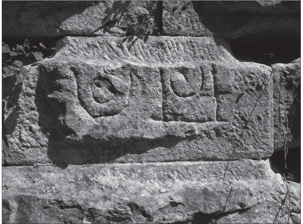
Fig. 6 Metamorphosed limestone facing stone with mason's mark from the 5 th -century aqueduct bridge of Kumarlıdere. – (Photo R. Snyder).
