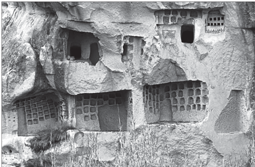
Fig. 2 Dovecotes on the front of rock-hewn dwellings in Göreme/TR. In the Early and Middle Byzantine Era many churches and large dwelling complexes were built into the tuff mountains of Cappadokia. Partially these have multiple storeys and are dozens of meters deep. They also comprise facilities like mills and stables. – (After Germanidou, Dovecotes 45 fig. 9).
