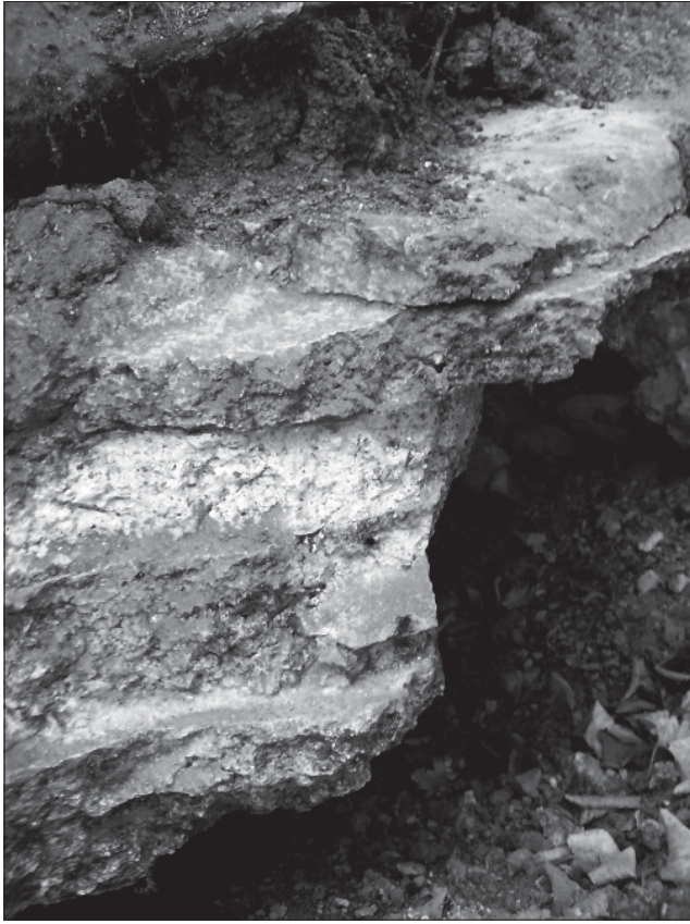
Fig. 10 Channel lining mortar in situ showing multiple events of re-plastering. – (Photo R. Snyder).
