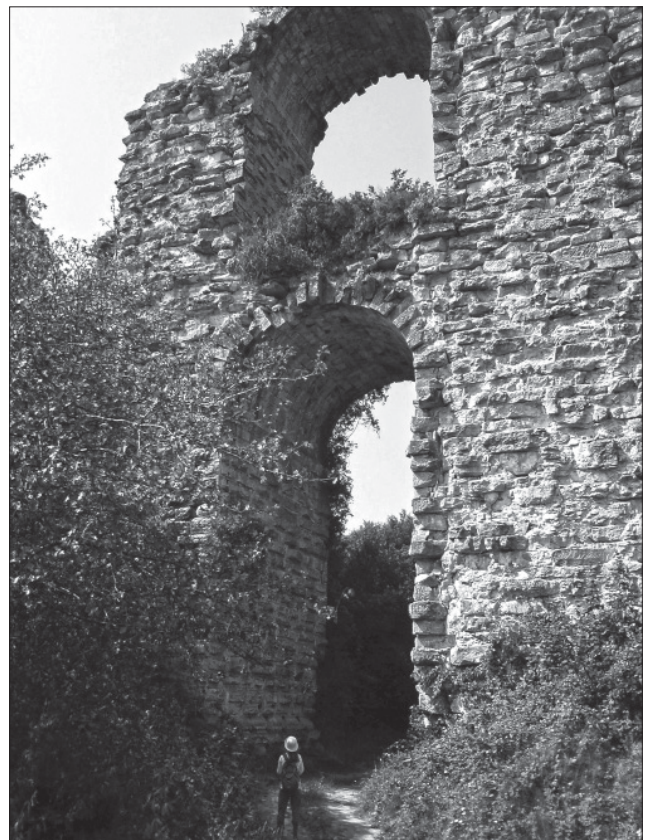
Fig. 7 5 th century aqueduct bridge of Kumarlıdere with exposed mortar and rubble core. – (Photo R. Snyder).
