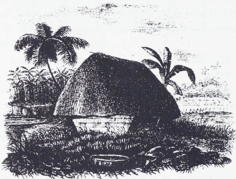
Fig. 23 A fale okofale ufi (storage house). Note the receding walls and the overhanging roof. This type of houses was reported by COOK and his officers as frequently occurring on Nomuka. The German caption of this French lithograph indicates that the house was drawn on Tongatapu. (Drawing by L. de SAINSON in 1826, on DUMONT d'URVILLE's first voyage to Tonga; this figure reproduced from the German edition).
