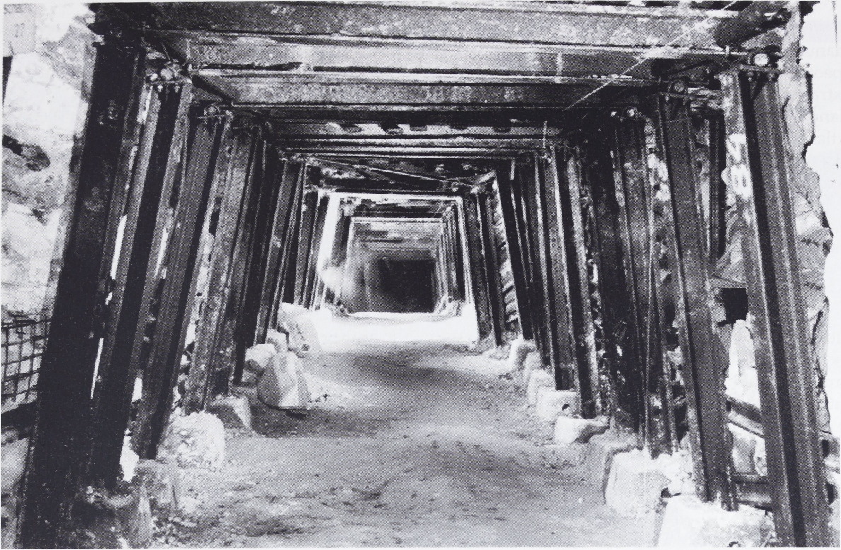
Fig. 12 The modern tunnel dug right across the prehistoric mining area after having been secured with steel supporting props.
