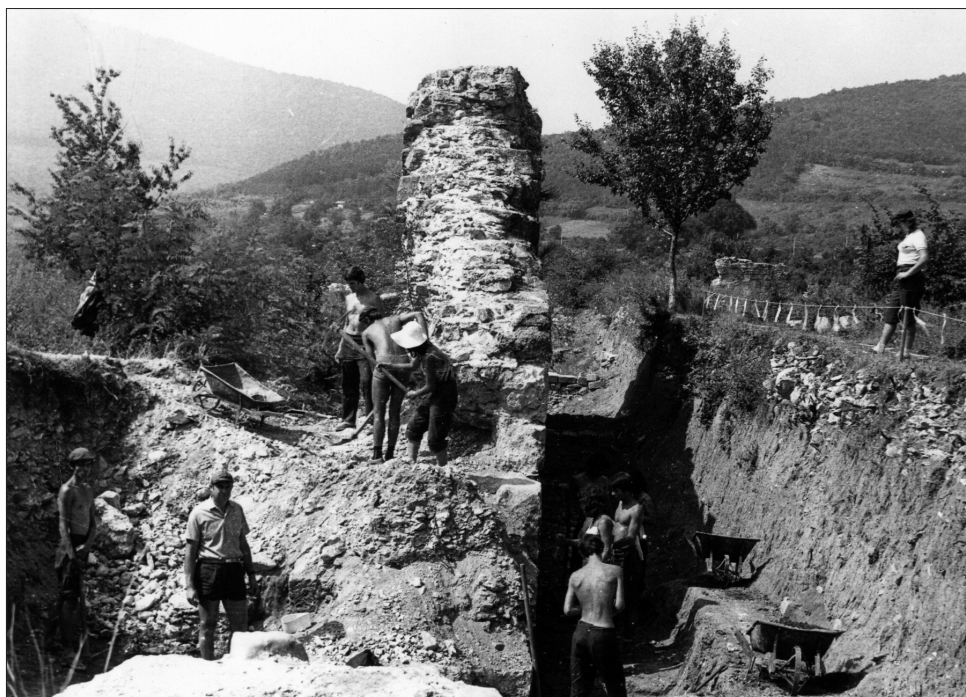
Fig. 8 The east fortress of the palace complex. – (Photo Archive of NAIM-BAS).
