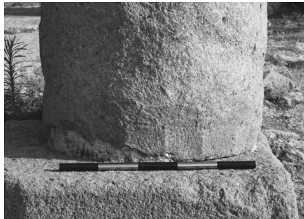
Figure 4 Pergamon, propylon of the Demeter sanctuary, unfinished twenty-sided polygonal column.
