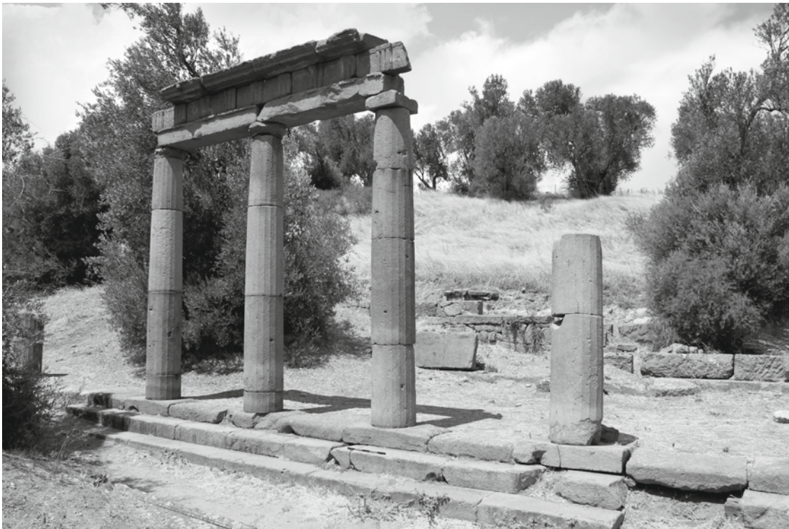
Figure 8 Pergamon, stoa west of the Asklepieion, twenty-sided polygonal columns with a slightly fluted necking of the capital.
